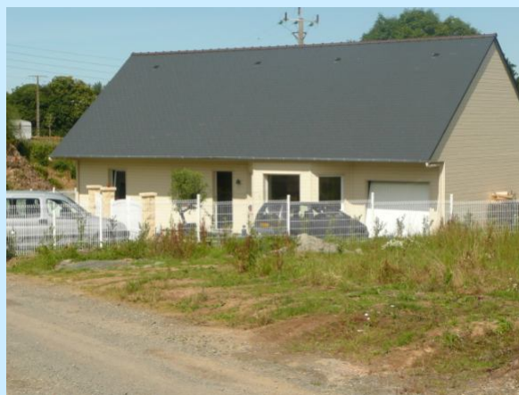
Construction neuve Park Ker An Run
